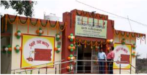
Figure 7 Hybrid Toilet inaugurated under BeMC to make the city ODF
