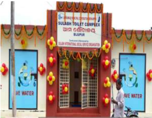
Figure 4 Hybrid Toilet inaugurated under BeMC to make the city ODF
