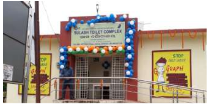
Figure 6 Hybrid Toilet inaugurated under BeMC to make the city ODF
