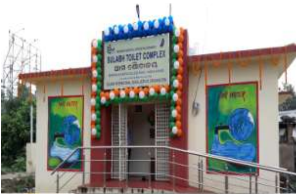
Figure 2 Hybrid Toilet inaugurated under BeMC to make the city ODF
